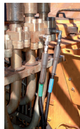
6 Load sensors to know the lifting pressure
